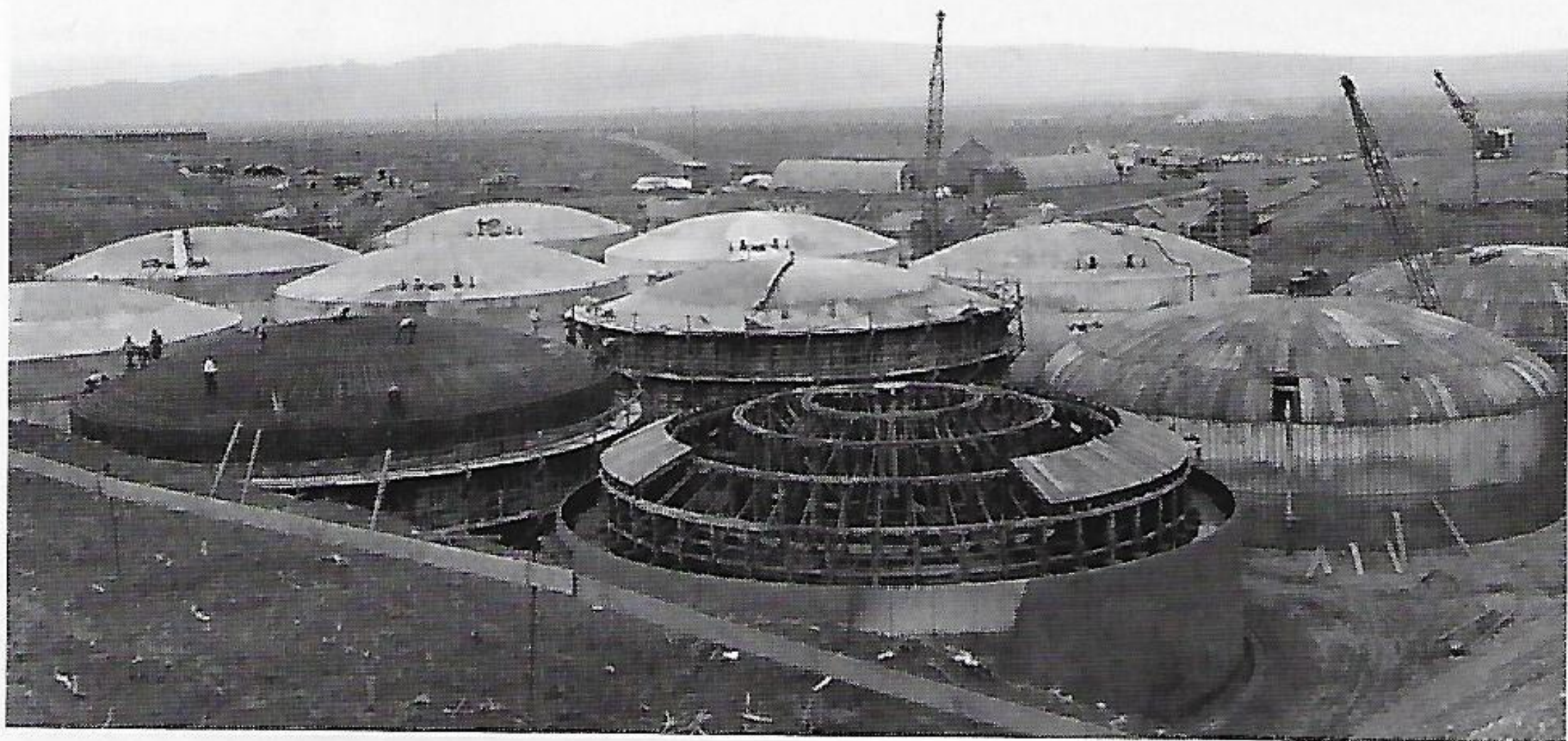
A tank farm on the Hanford reservation under construction
